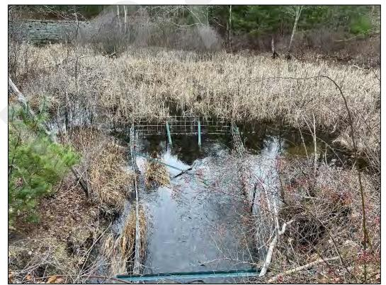
Photo No. 36.: Reach\_B\_#13 – Beaver deceiver installed upstream of the Putnam Hill Road culvert.
